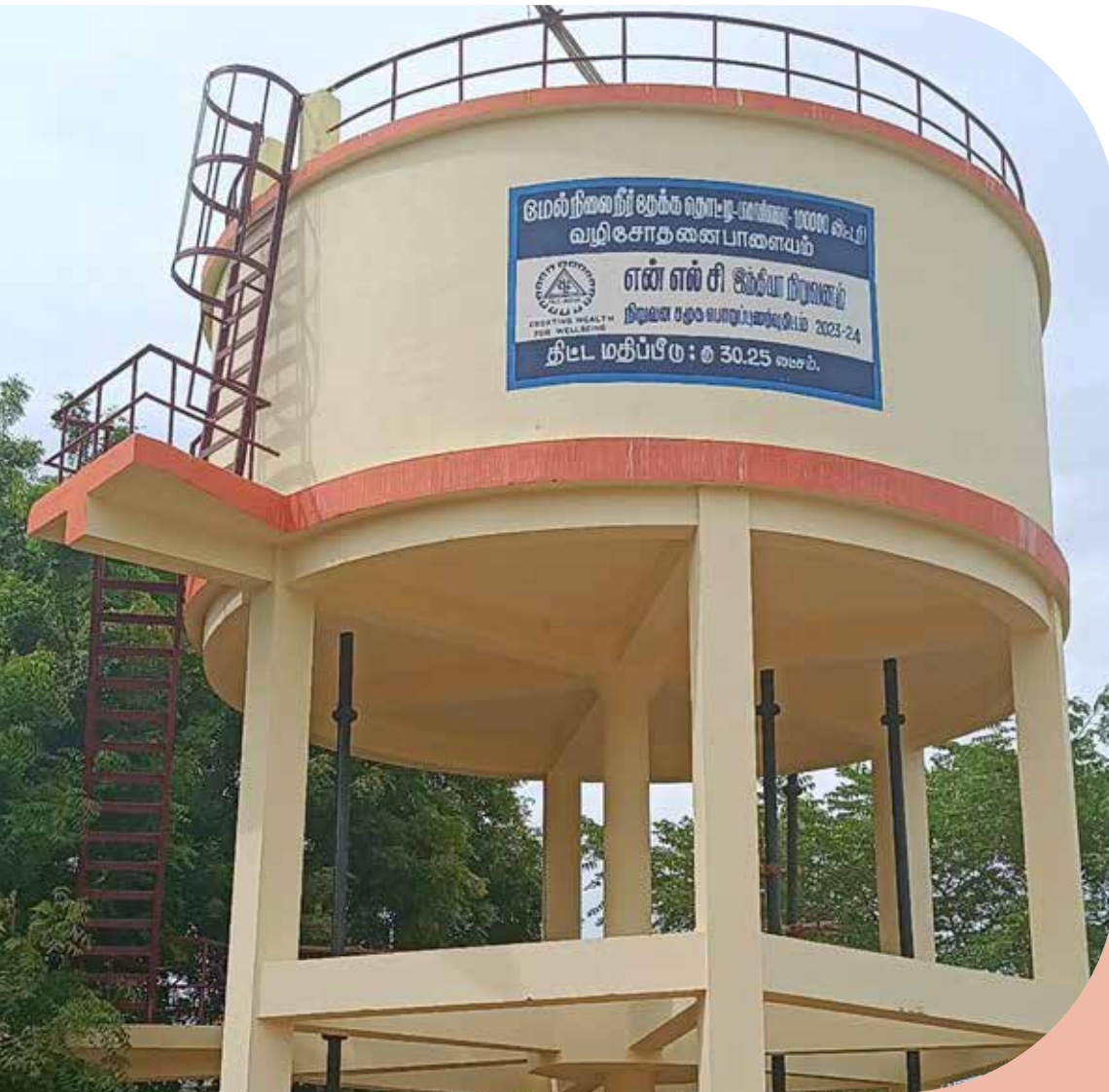
Construction of 1,00,000 Capacity OHT Tank at Annavalli Uratchi, Vazhisothanai Palayam Village
