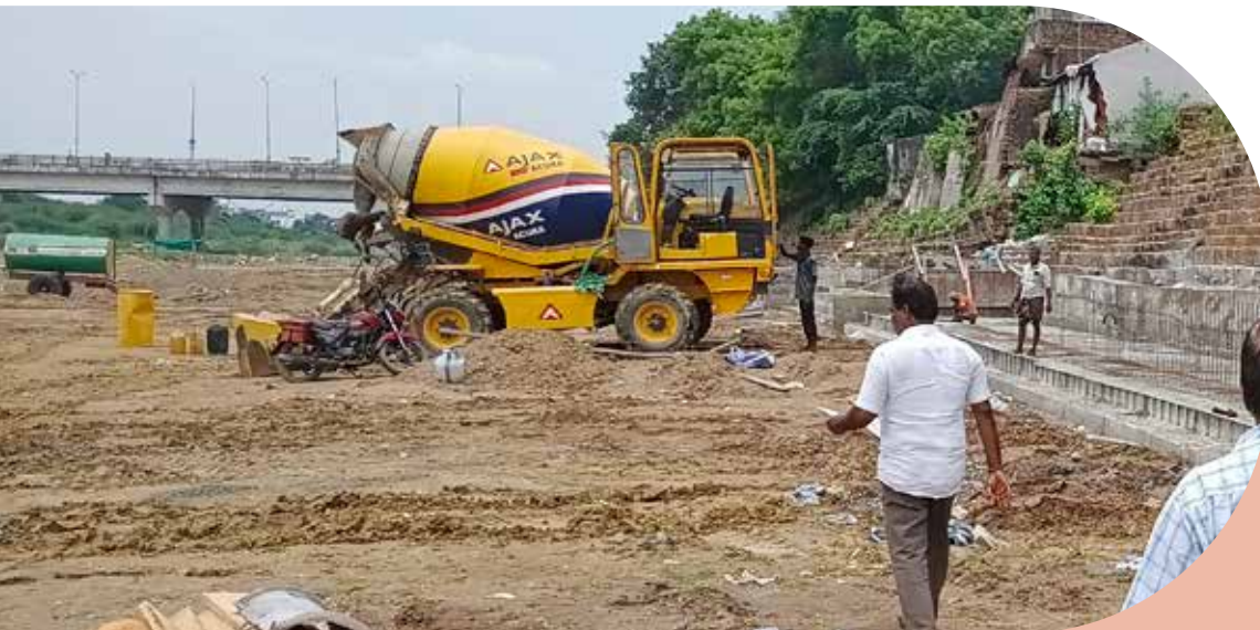
Restoration work of Manimuktharu River at Vridhachalam
