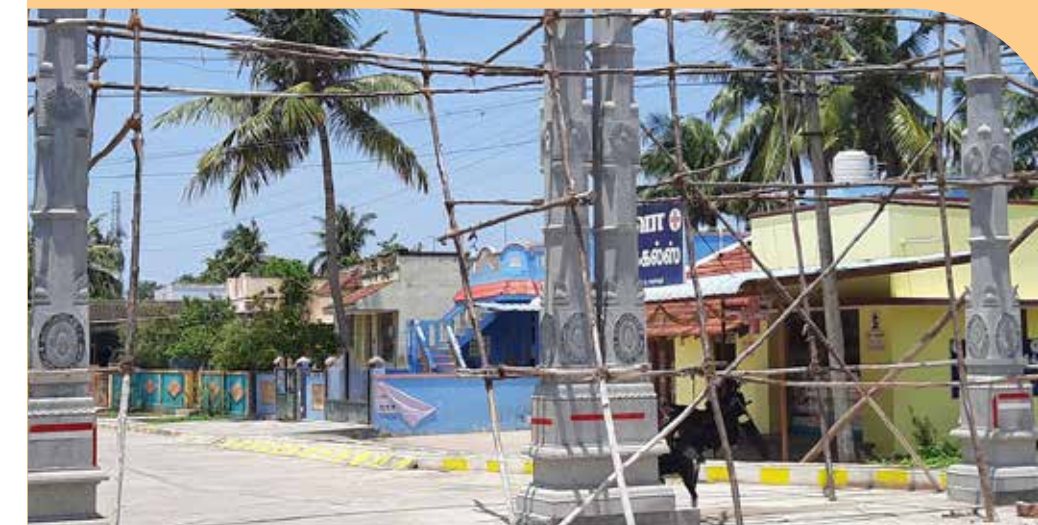
Providing CC Road with Pedestrian Walk to Reddiyar Street near Thanneeril Vilaketriya Illam in Karunkuzhi panchayat.
