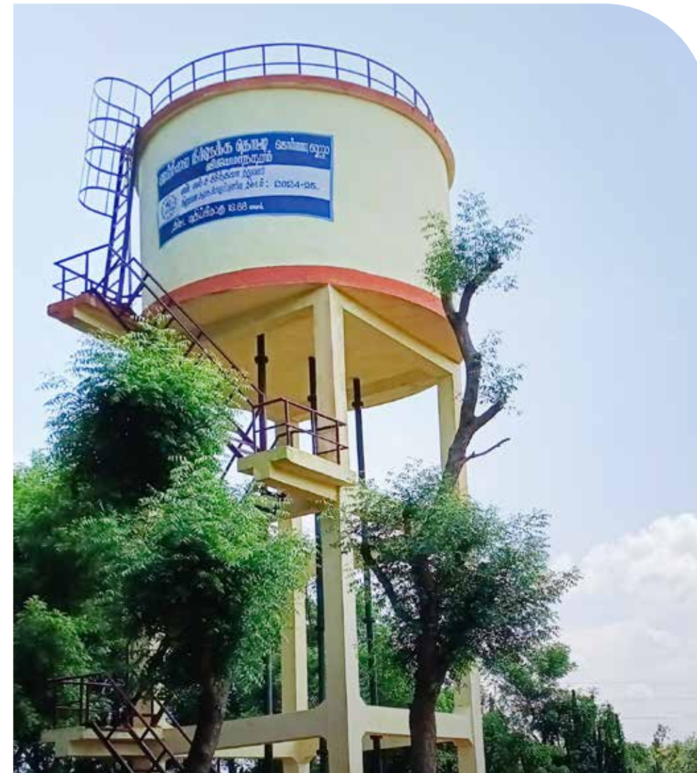
Construction of 60000 Lit capacity OHT in Vijayamanagaram Panchayat
