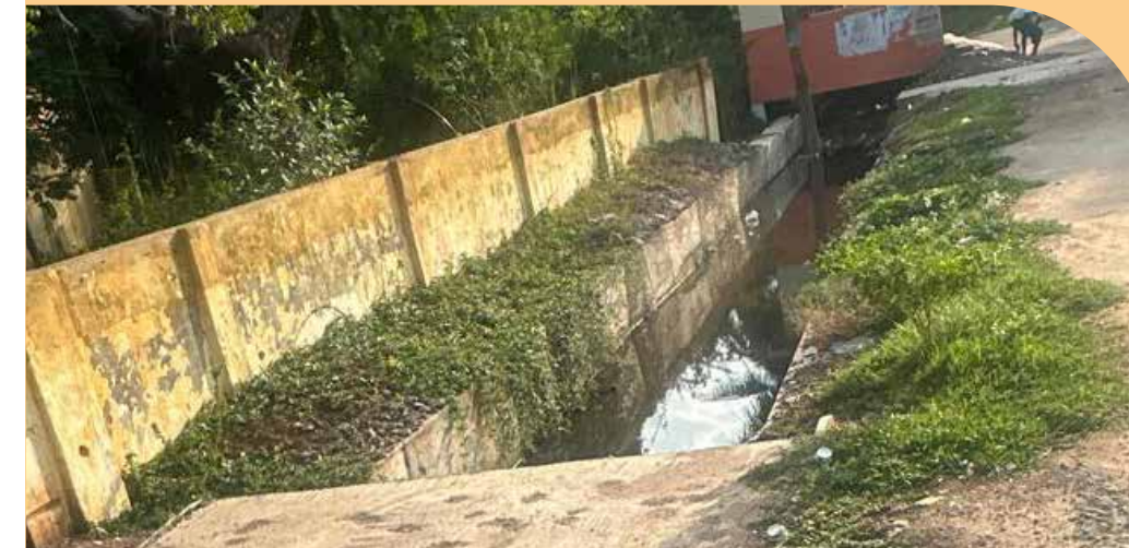
Construction of Drainage near Mettukuppam Sithivilagam Koil in Karunkuzhi Panchayat
