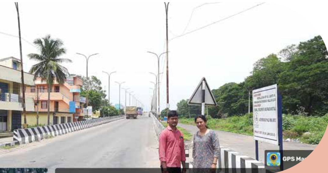
Installation of lights in Pennadam (Eraiur) Bridge
