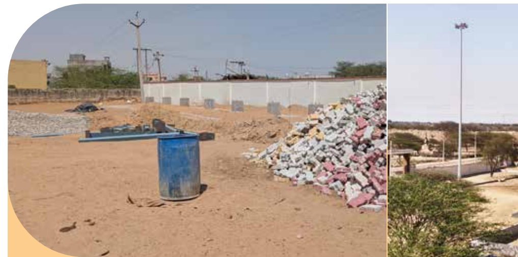
Infrastructure development at Community Health Center (CHC), Barsingsar
