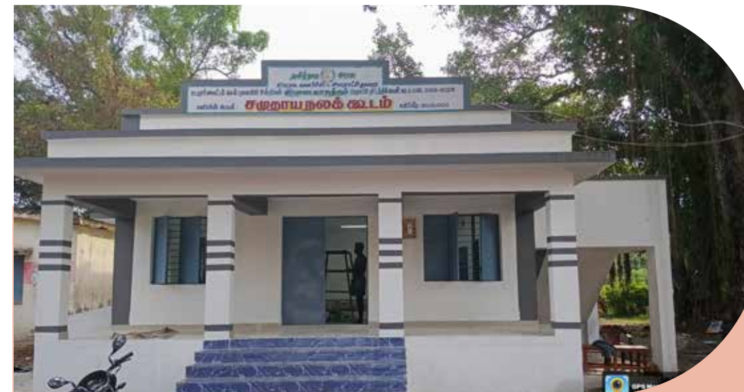
Construction of Community Hall at Veeramudaiyanatham in Melbhuvanagiri Block
