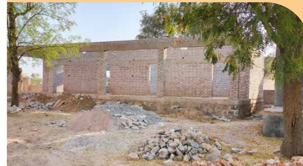
Infrastructure development at Govt. Sr. Sec. School, Swaroopdesar
