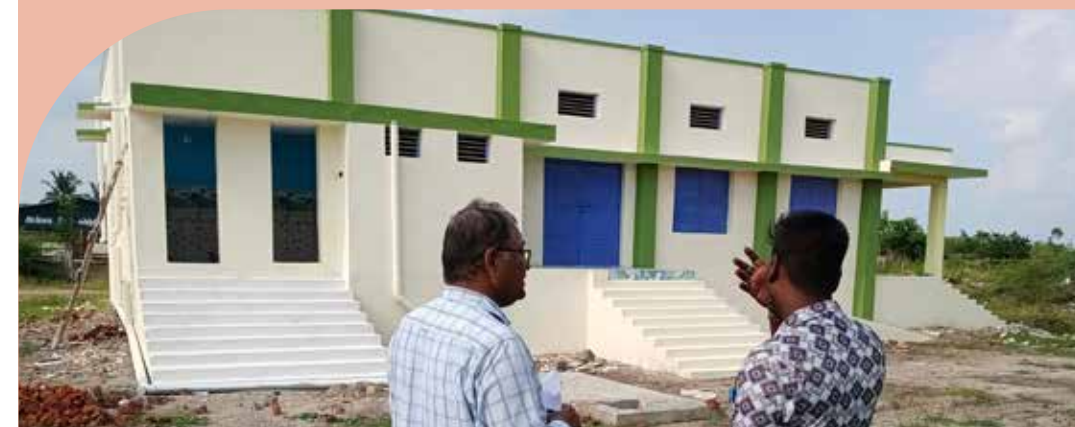
Construction of Community Hall at Kammapuram in Kammapuram Block
