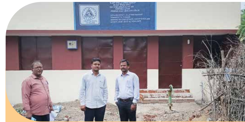
Construction of Anganwadi Building at Killai Town Panchayat
