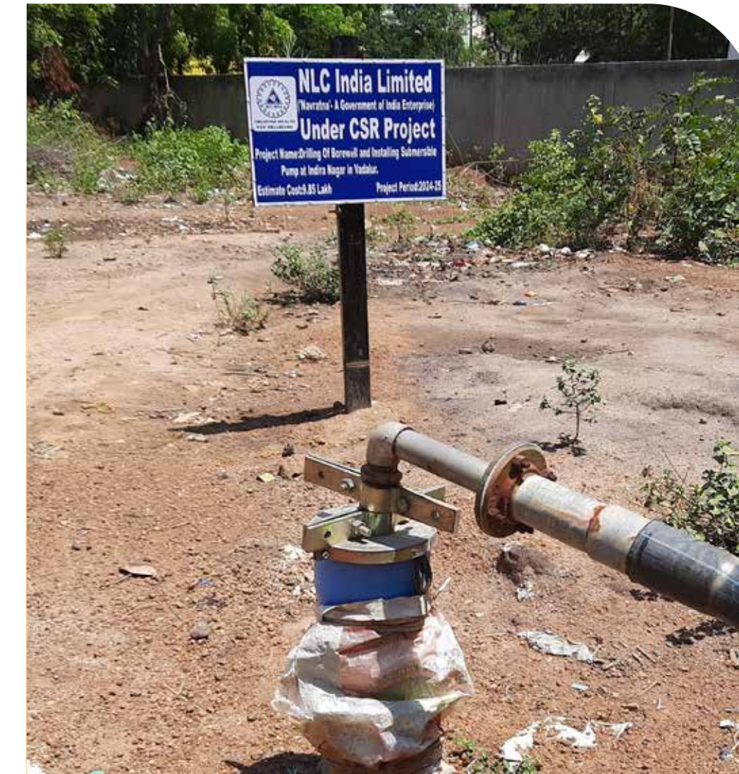
Revitalisation/Drilling of Borewell at Vadalur Municipality (Indira Nagar, Maruthi Nagar) Drilling and installation of submersible pump at Indiranagar in Vadalur
