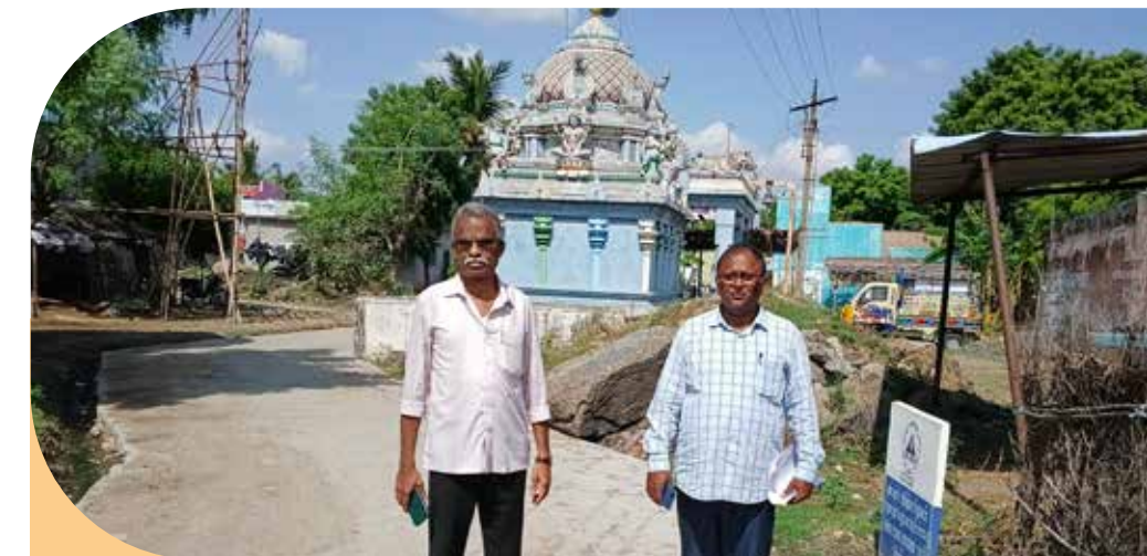
Construction of Cement Road in Kovilanur Panchayat - 200 Meter
