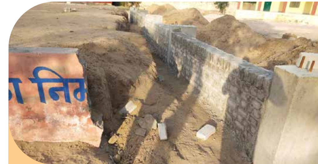
Construction of shade for wrestling ground in Mahatma Gandhi school, Barsingsar
