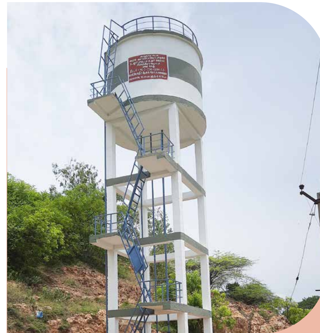
Construction of OHT (30,000 Ltr) at Malaisanthu, Thiruvanthipuram Panchayat in Cuddalore block
