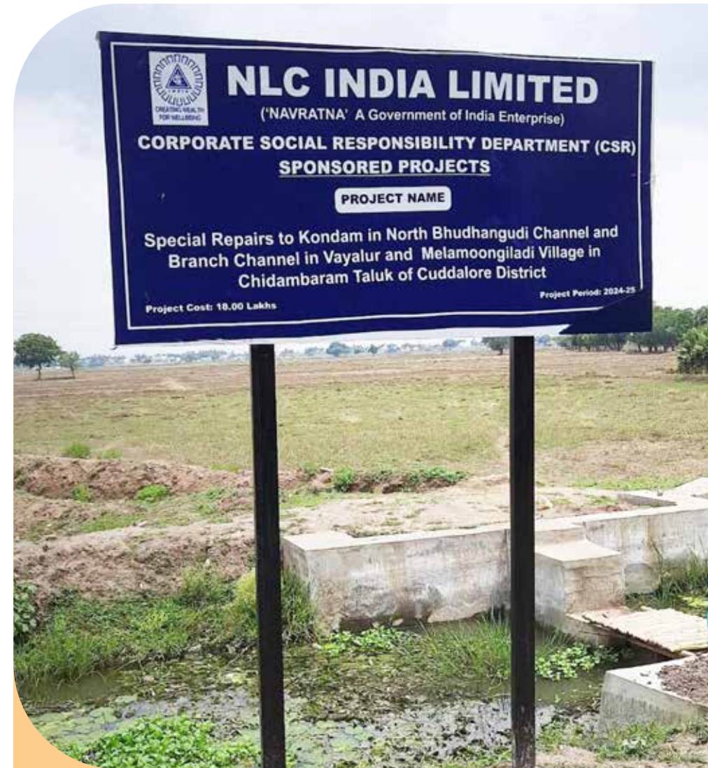
Special repairs to Kondam in North Bhudhangudi channel and branch channel in Vayalur and Melamoongiladi Village in Chidambaram Taluk
