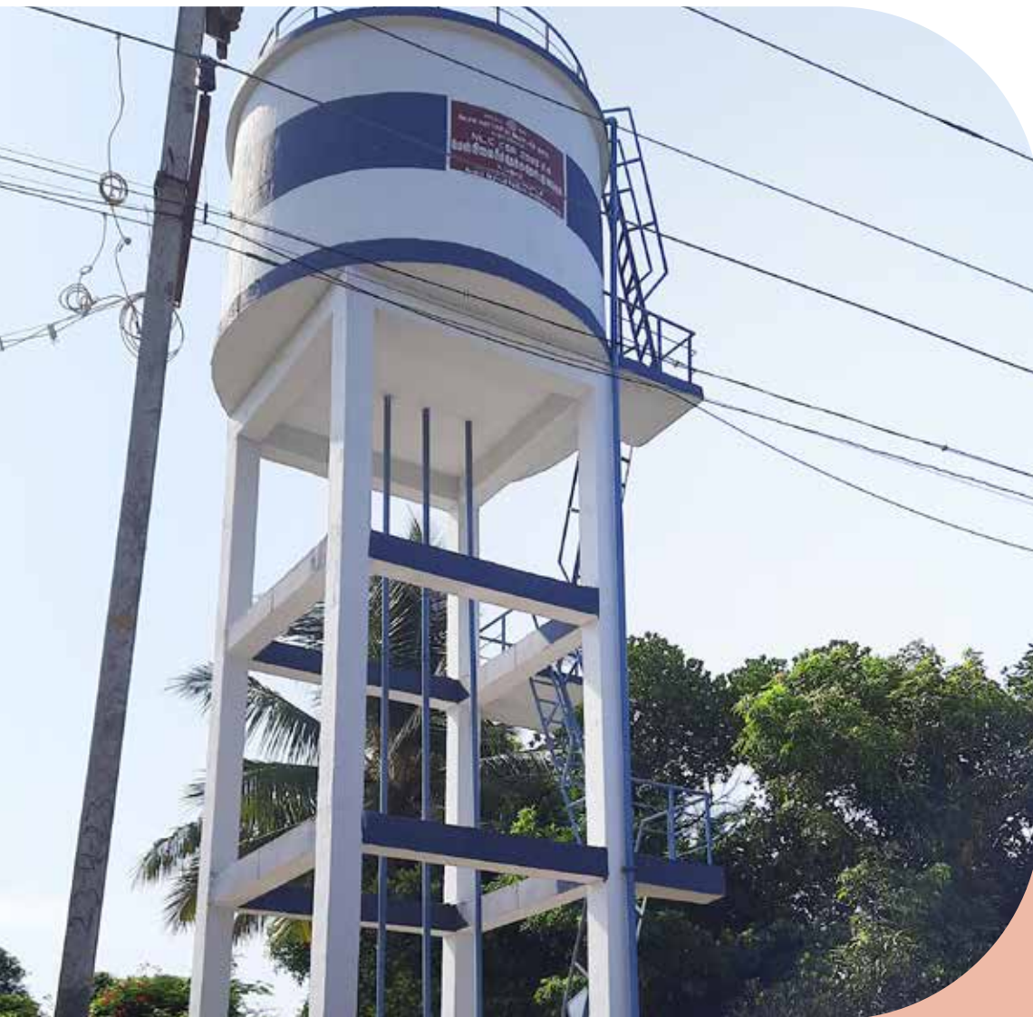
Construction of OHT (30,000 Ltr) at K. Pudur, Karaikadu Panchayat in Cuddalore block
