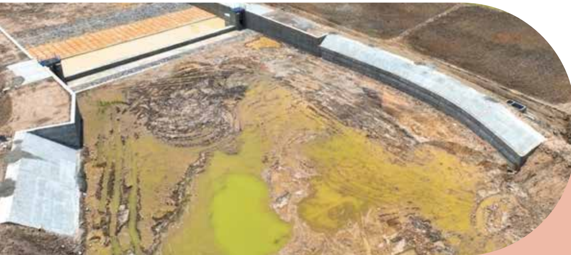
Comprehensive flood protection works to the Peria Odai from Wellington Reservoir surplus course to confluence point in Kazhudhur Odai near Sirumalai Village in Tittakudi Taluk of Cuddalore District
