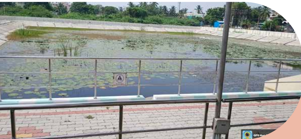
Providing paver walkway and lining work inside pond at Swamy Sagajanantha Mani Mandapam at Chidambaram
