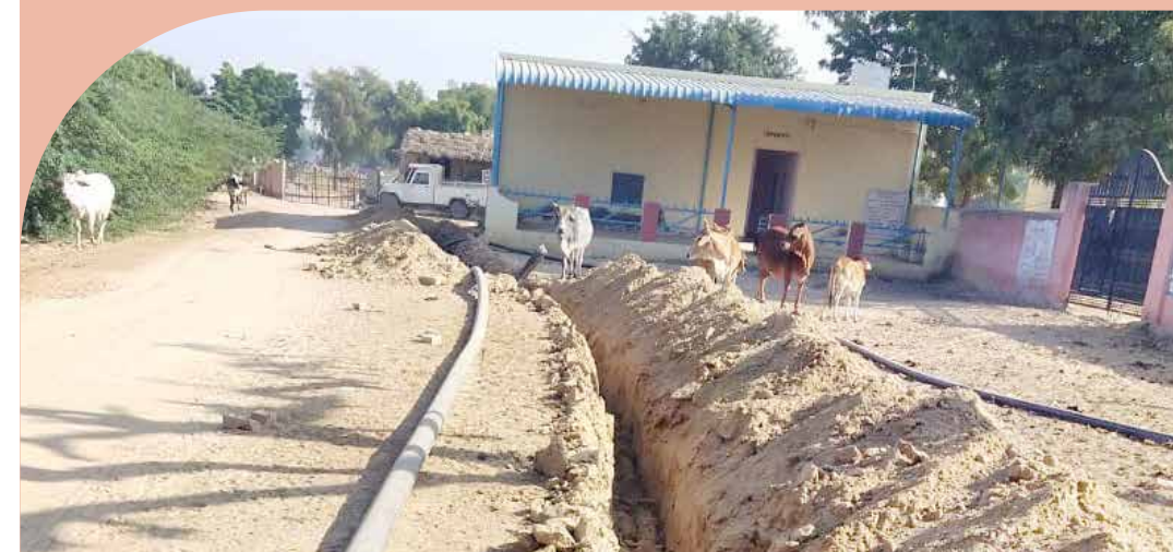
Shifting of water supply lines at Swaroopdesar village
