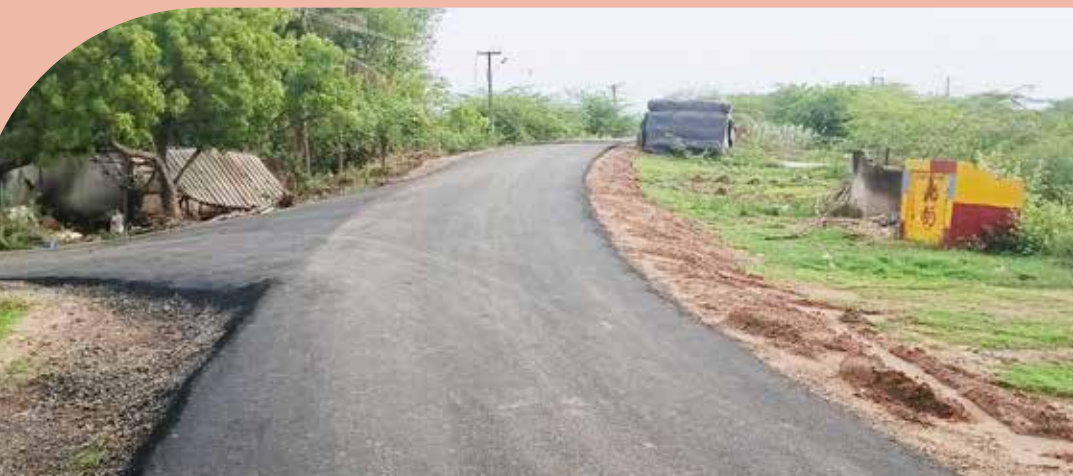
Laid out 4.8 Km link road from VKT road to Thiruvannainallur (Antharasipettai) at Kalkunam Panchayat, Kurinjipadi Block
