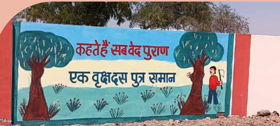
Renovation of Boundary wall in Govt. Primary school Basi (North)
