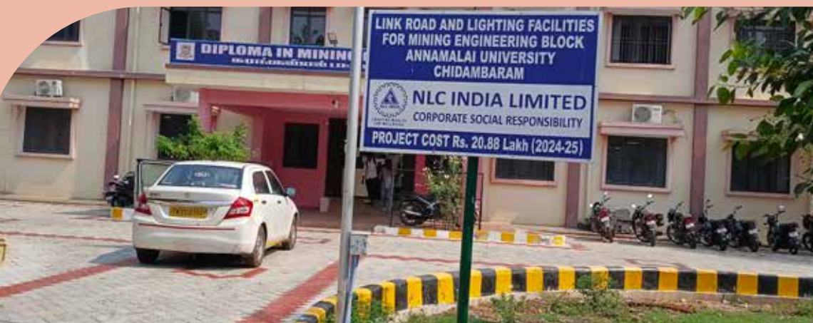
Providing link road with paver blocks including lighting facilities for Mining Engineering block at Annamalai University
