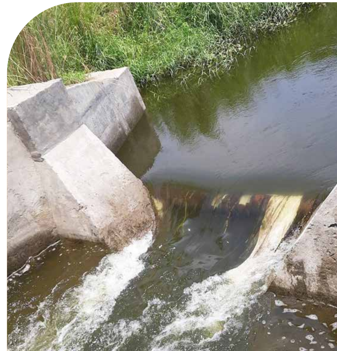
Rehabilitation of Vandurayanpattu Notch across Manampathan Channel at Vandurayanpattu Village in Bhuvanagiri Taluk
