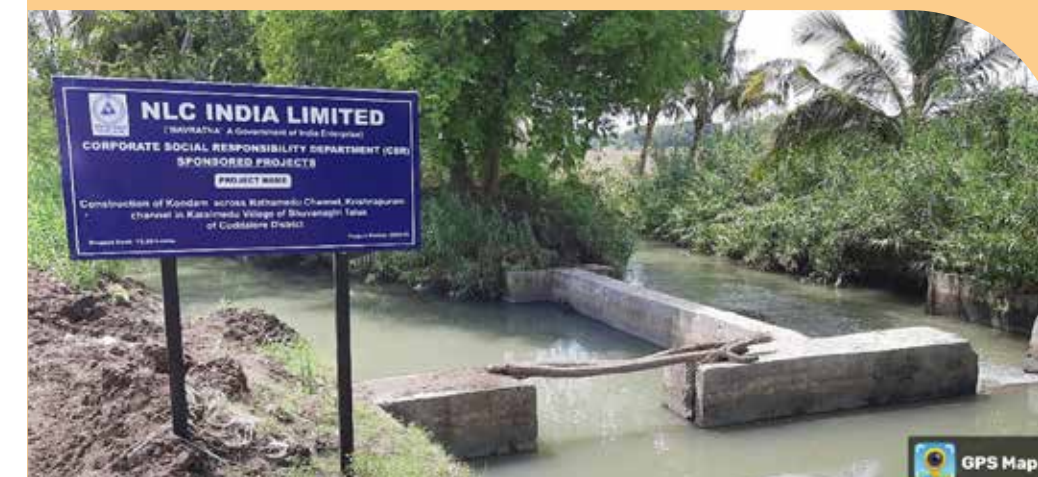
Construction of Kondam across Nathamedu Channel, Krishnapuram Channel in Karaimeadu Village of Bhuvanagiri Taluk
