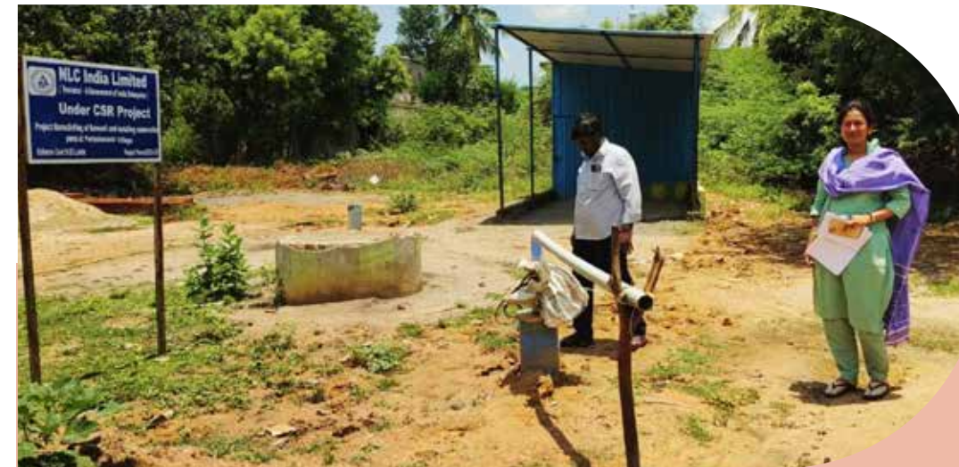
Drilling of borewell & installation of submersible pump at Periyakuruchi village
