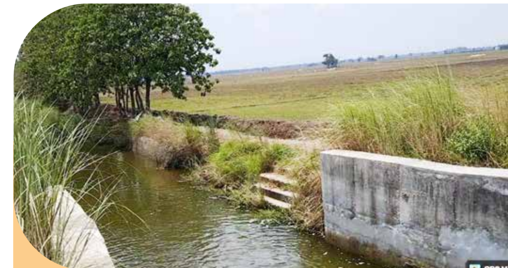
Special Repairs to Udayur Kondam in Udayur Village of Bhuvanagiri Taluk
