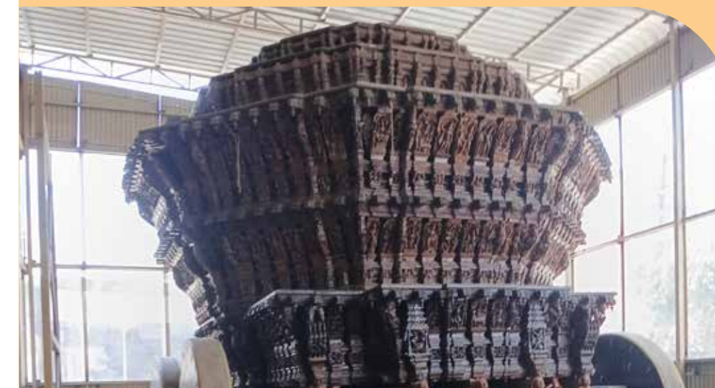
Construction of new transparent sheds for Chariots at Shri Sabanayagar Temple in Chidambaram
