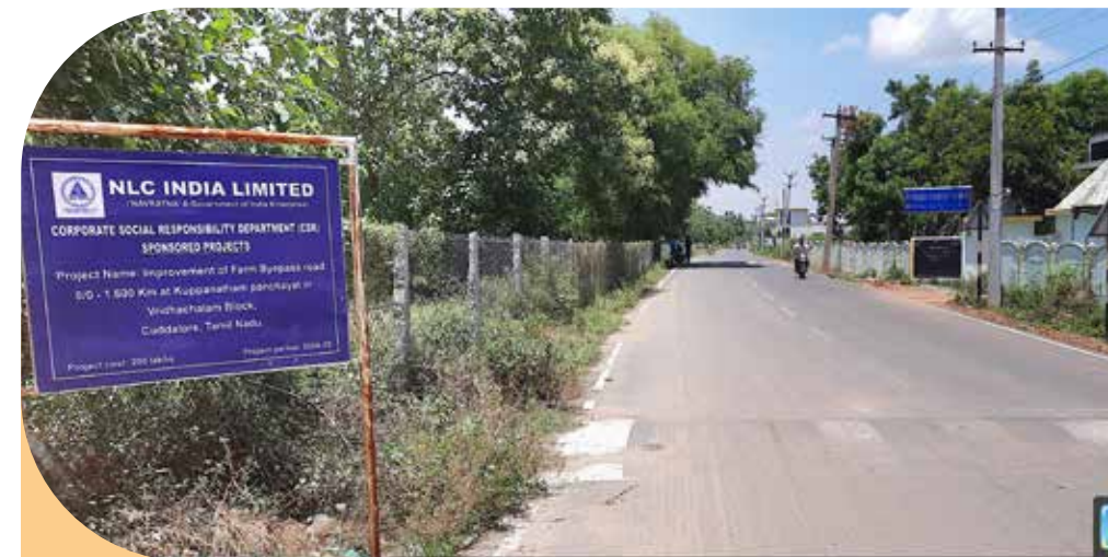
Development of Farm Bypass road 0/0 - 1/600 at Kuppanatham Panchayat in Vridhachalam Block
