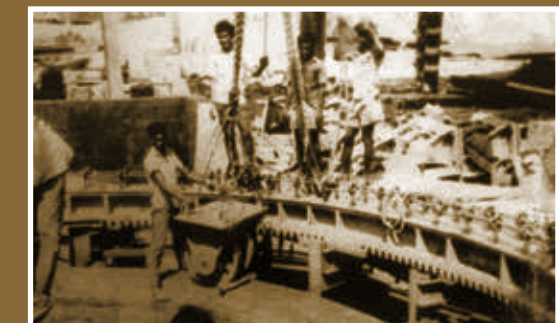
Erection of bath rotation wheel
