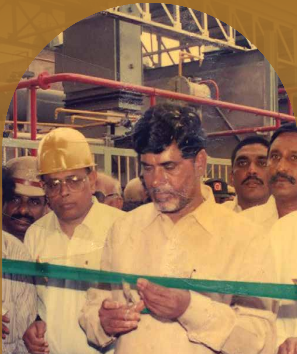
Inauguration of Power Plant at Paloncha by the Hon'ble Chief Minister of the then united Andhra Pradesh, Sri N Chandrababu Naidu
