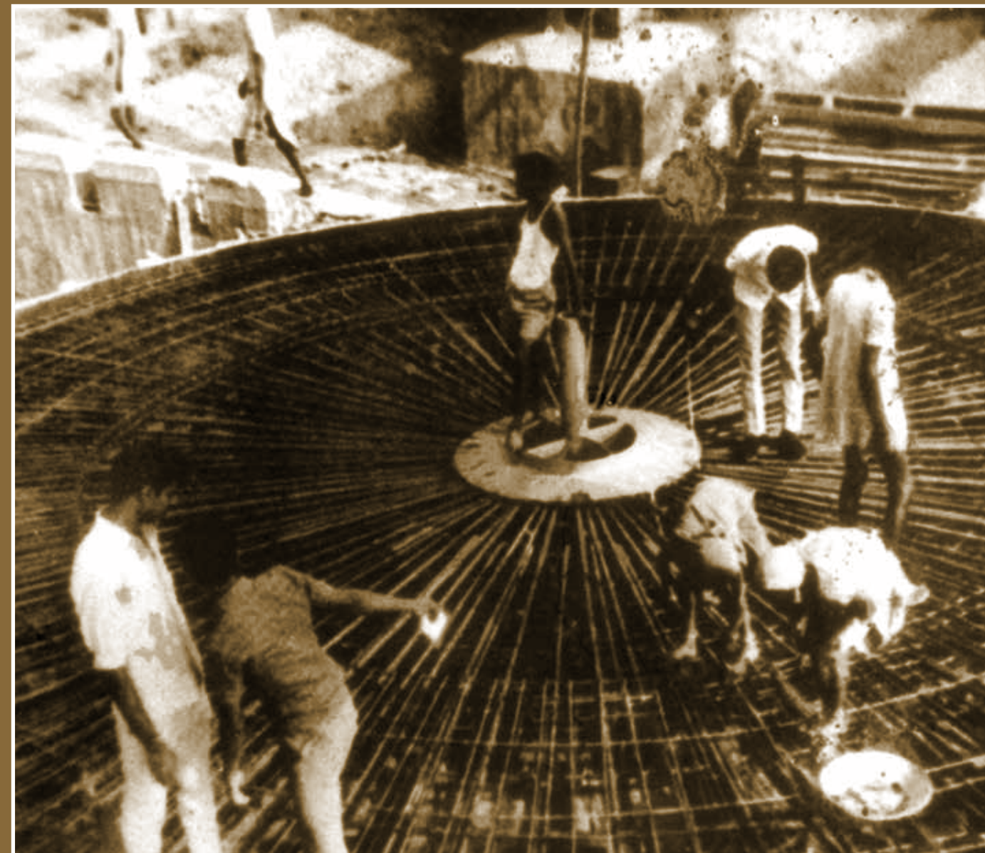
Erection of furnace bottom
